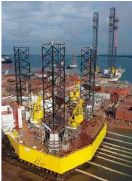
The jack-up rig Perro Negro 6 on the slipway at DDW's Graha Shipyard on Batam Island, Indonesia
